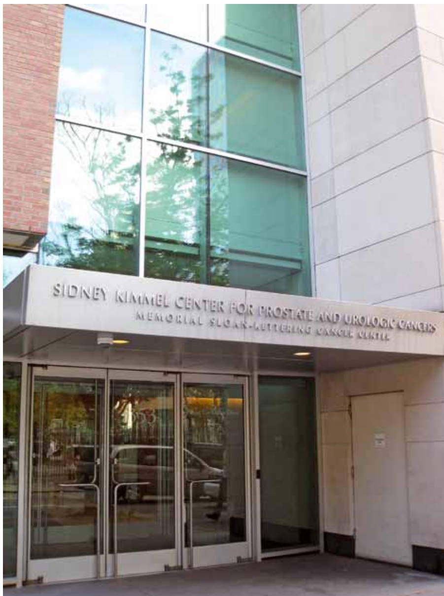
Main entrance of the MSKCC Sidney Kimmel Building
